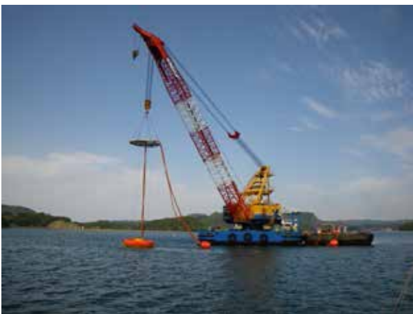
Photo-1 Set SMC to the crane barge
