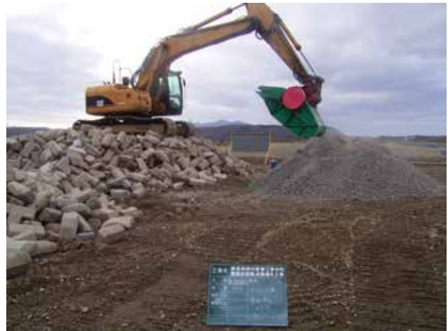
Picture 2, Producing Crusher Run On Site
